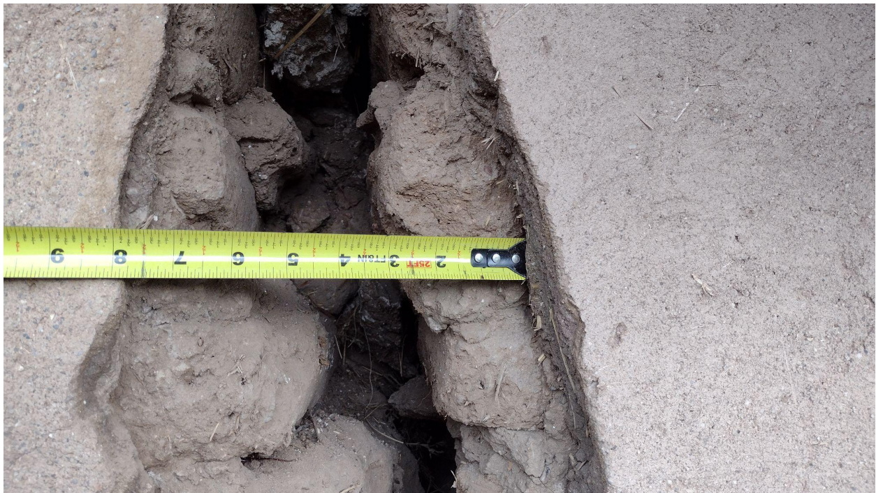
Separation of adobe bricks at union of new and old wall
