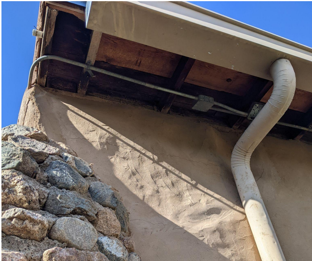
Final layer of plaster on northeast corner of wall
