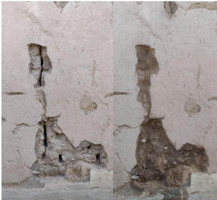
Left: Before crack repair and filling Right: after repair
