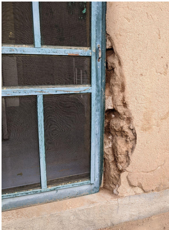
Loose material around door is removed (compare with next photo)
