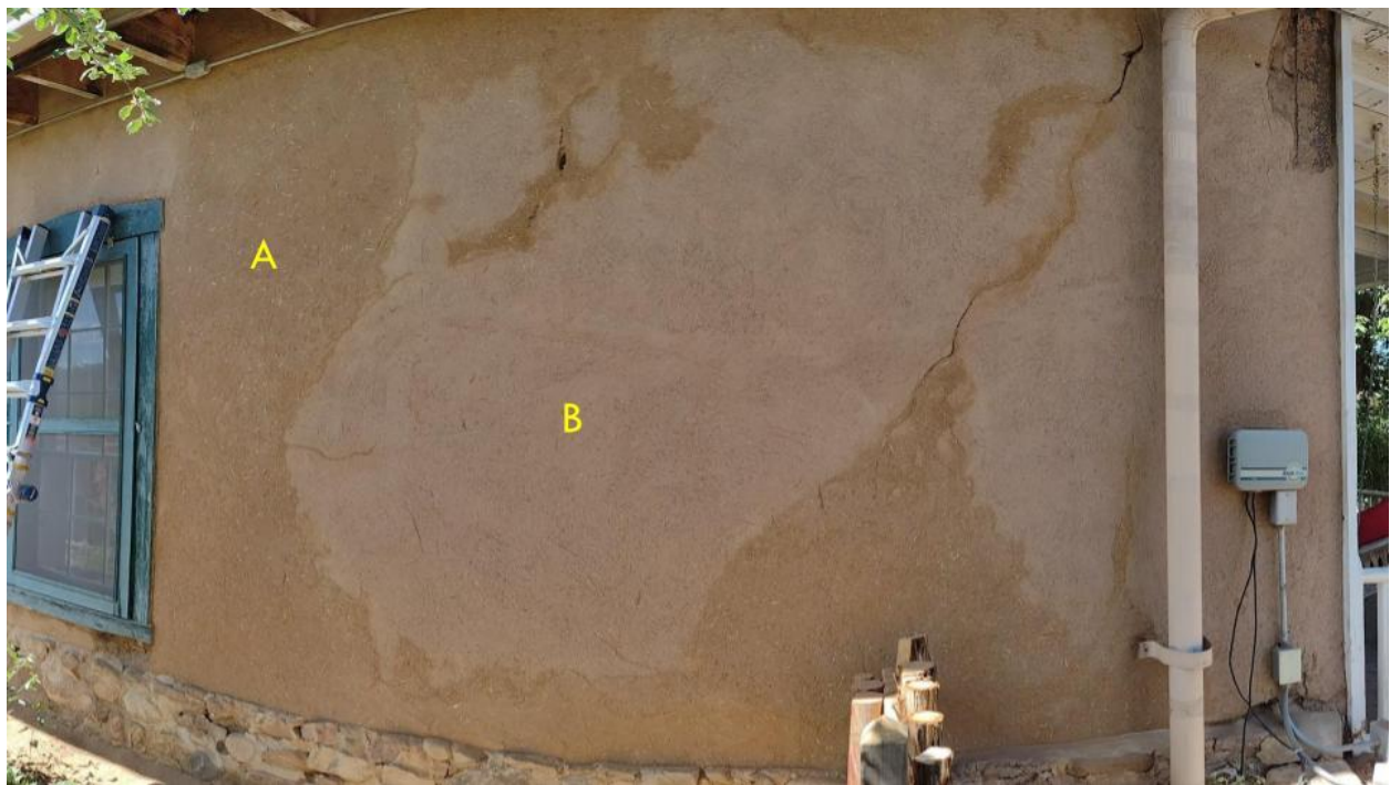
A: newer patchwork of repair plaster, B: older layer of pink-hued mud
