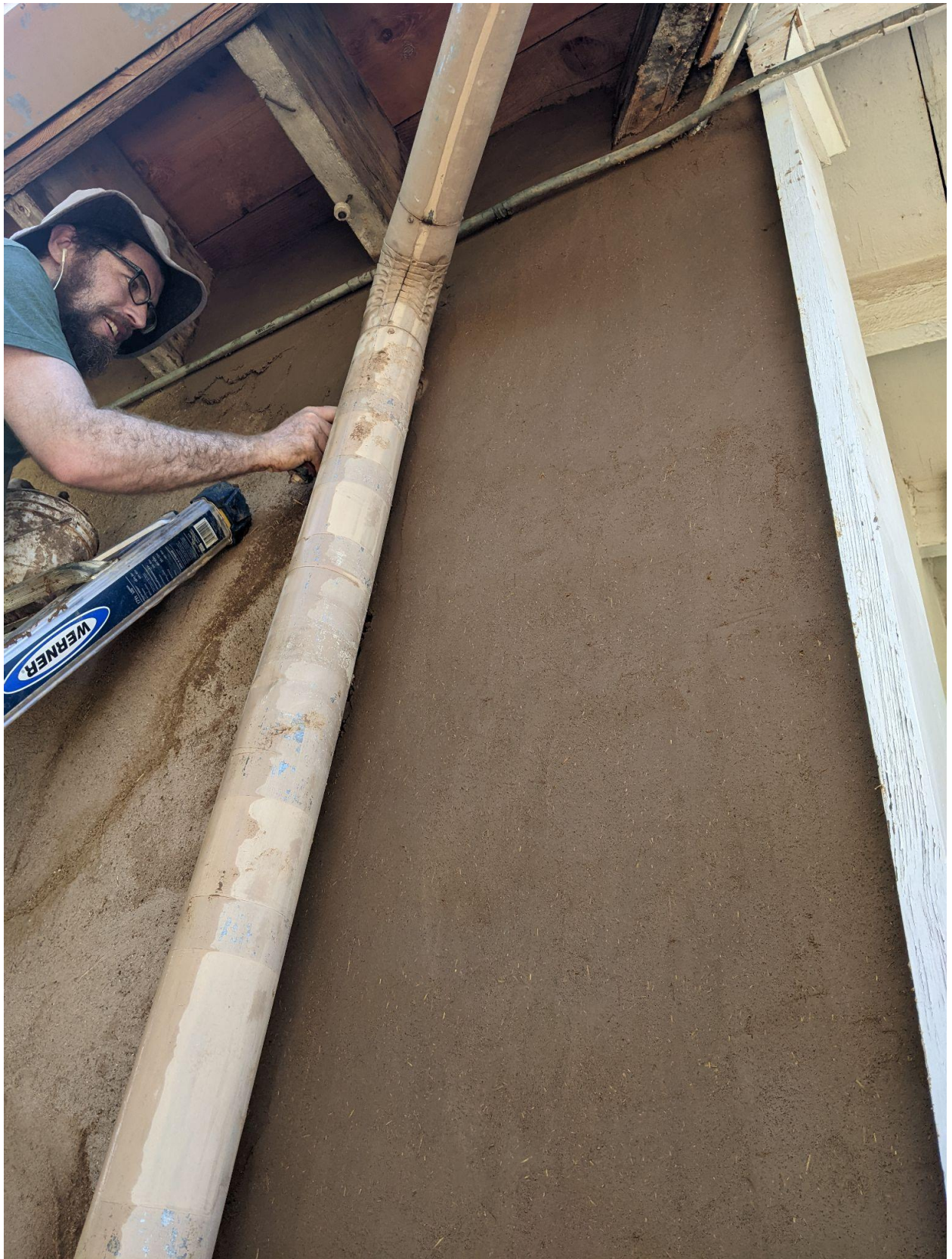
When the plaster is freshly applied, the straw contrasts with the damp clay
