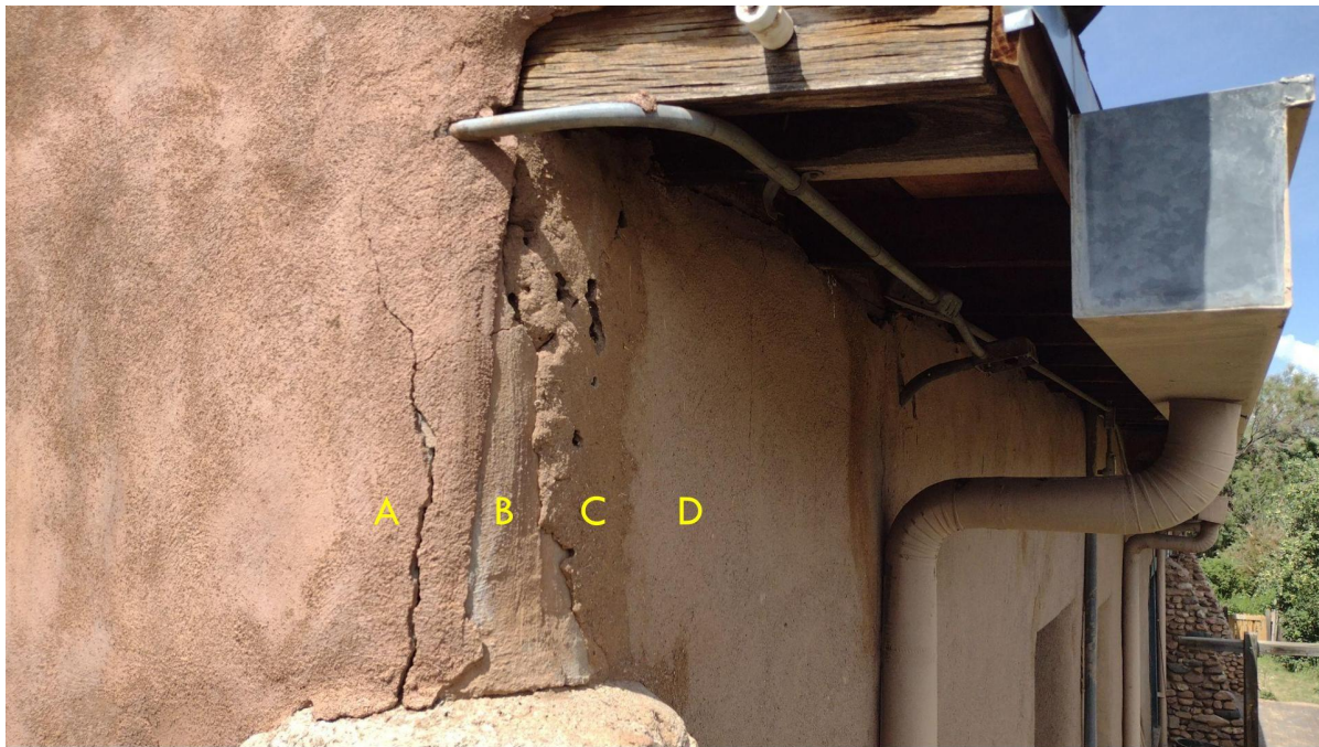
A: Modern stucco plaster, B: cement element, C: recent earthen plaster (note insect entries), D: 'pink' layer of plaster
