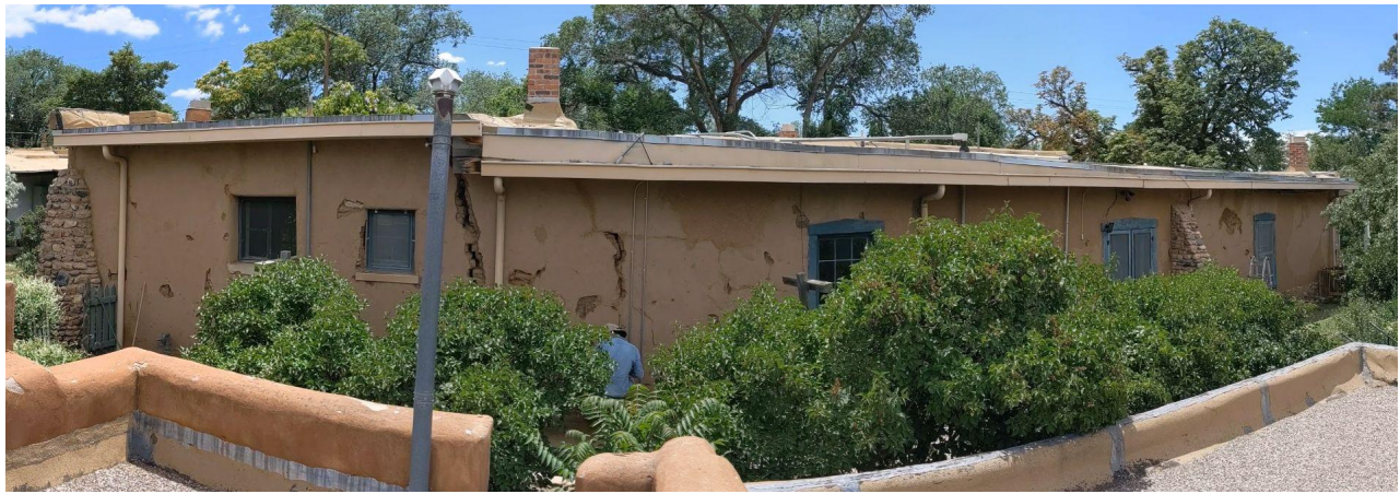
View of entire Northern wall during crack repair, before earthen plastering began
