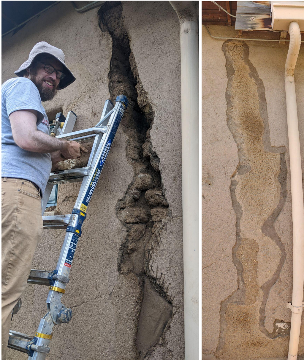
Left: Large gap between old and new wall is partially filled, Right: Gap has been fully patched
