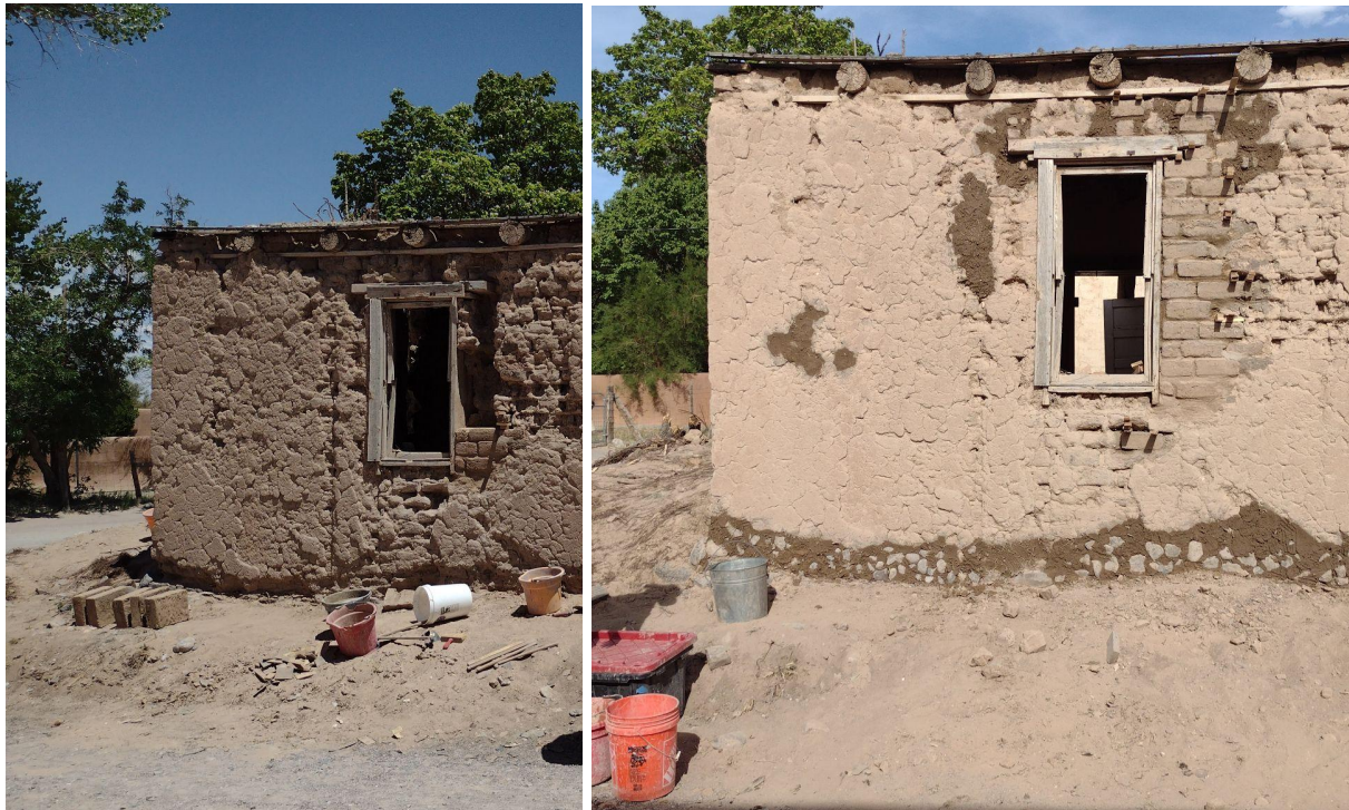
During and after a series of preservation treatments that addressed the eroded base of the wall, and the replacement of bricks on the side and above the window opening
