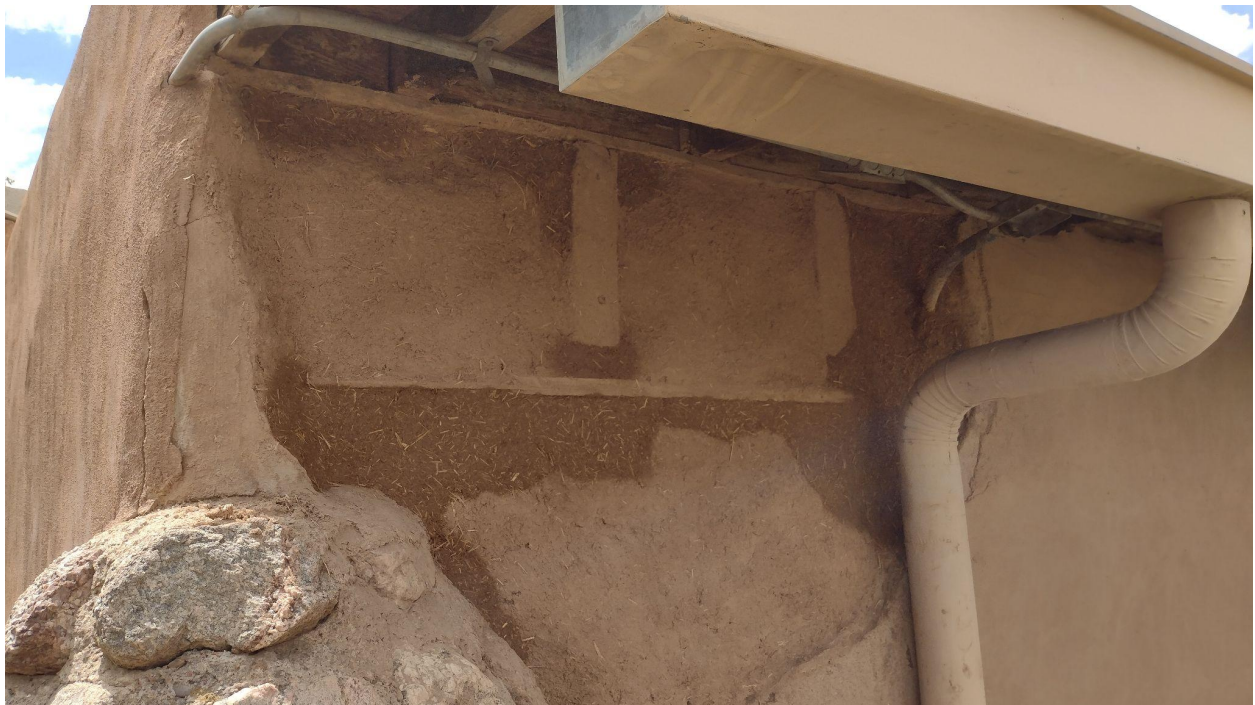
Corner area with voids filled with cob and initial layer of plaster covering wooden elements
