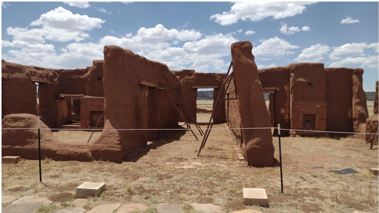
Structural stabilization of adobe walls that might otherwise benefit from having a roof system
