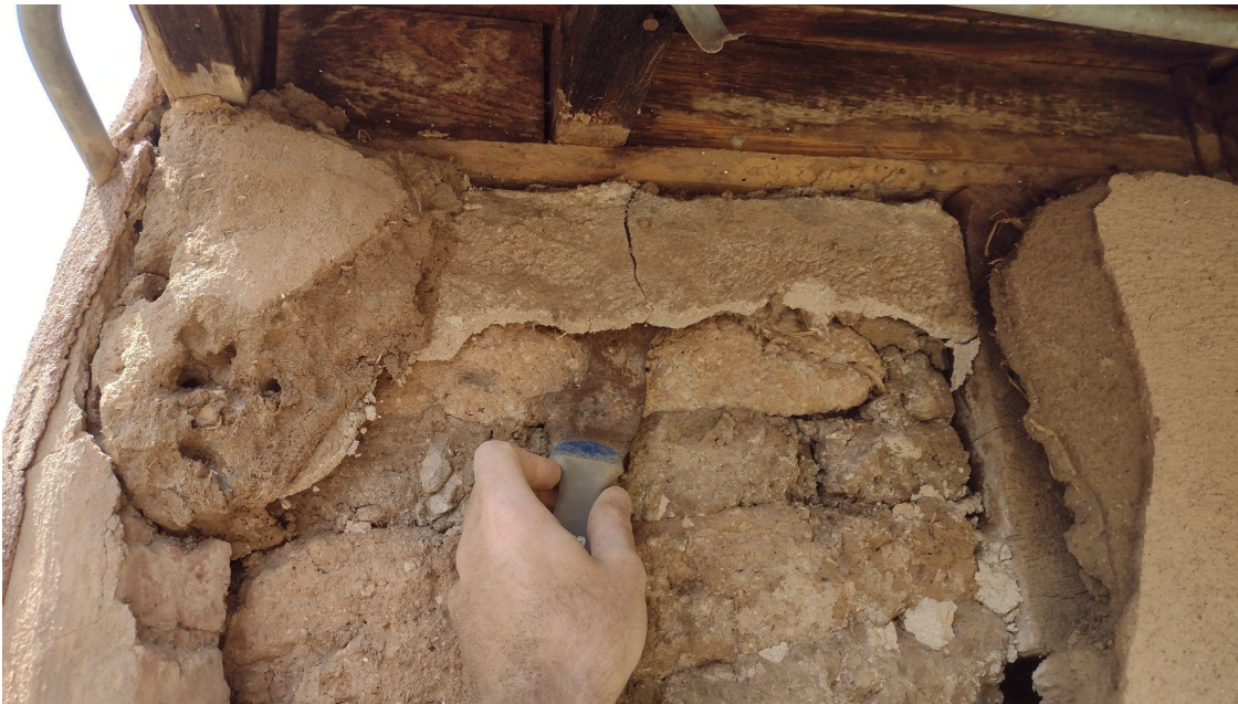
Removing layers of loose cement plaster
