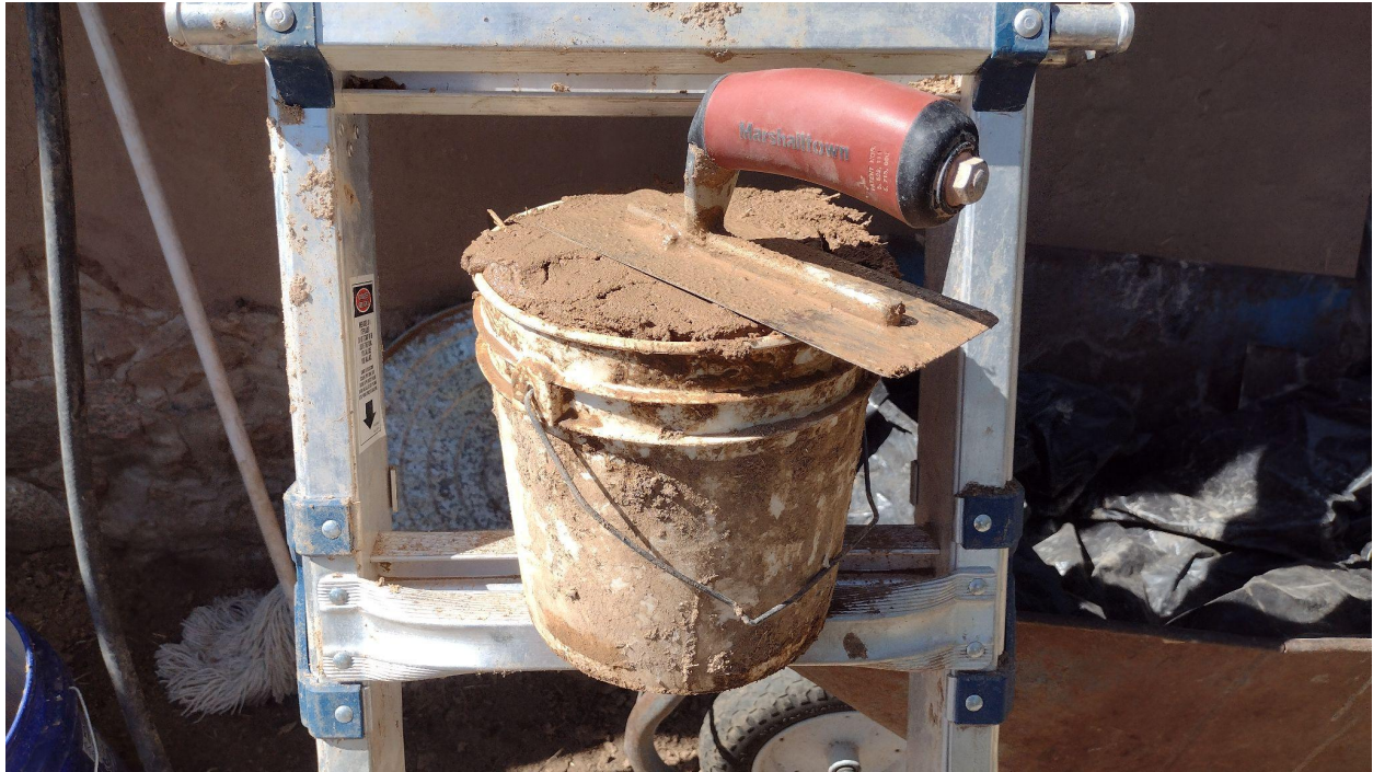
A gallon of prepared earthen plaster ready for application
