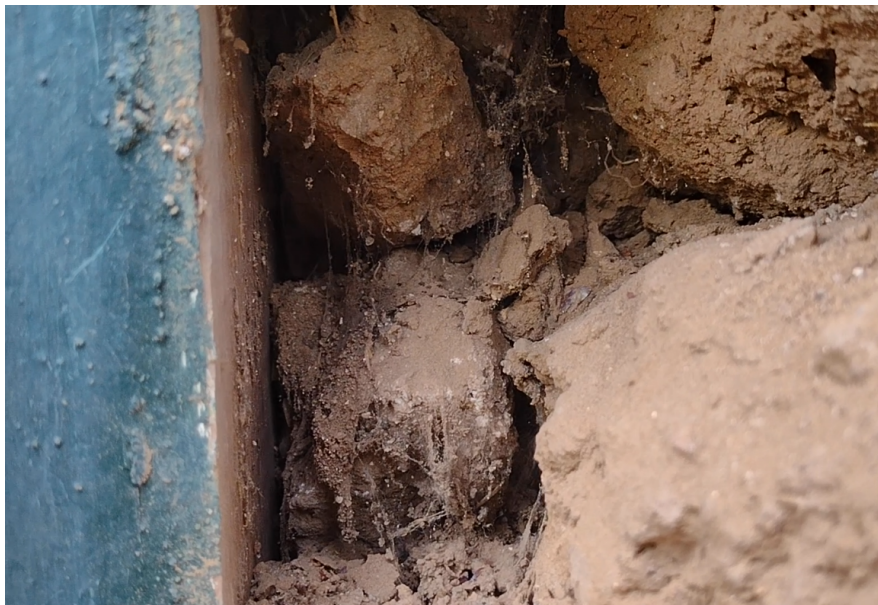
Example of area with loose/crumbled adobe bricks and presence of cobwebs
