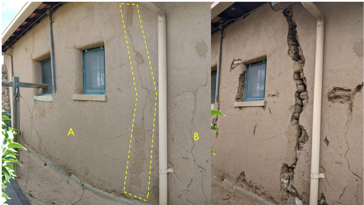
Before (left) and after (right) removing the plaster around the gap between the newer (A) and older (B) building
