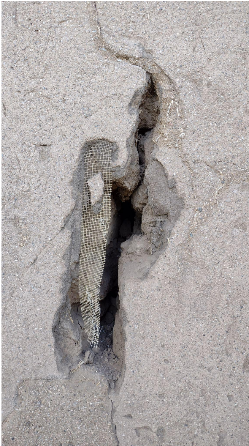
Use of drywall mesh tape used in previous repair efforts near large gap
