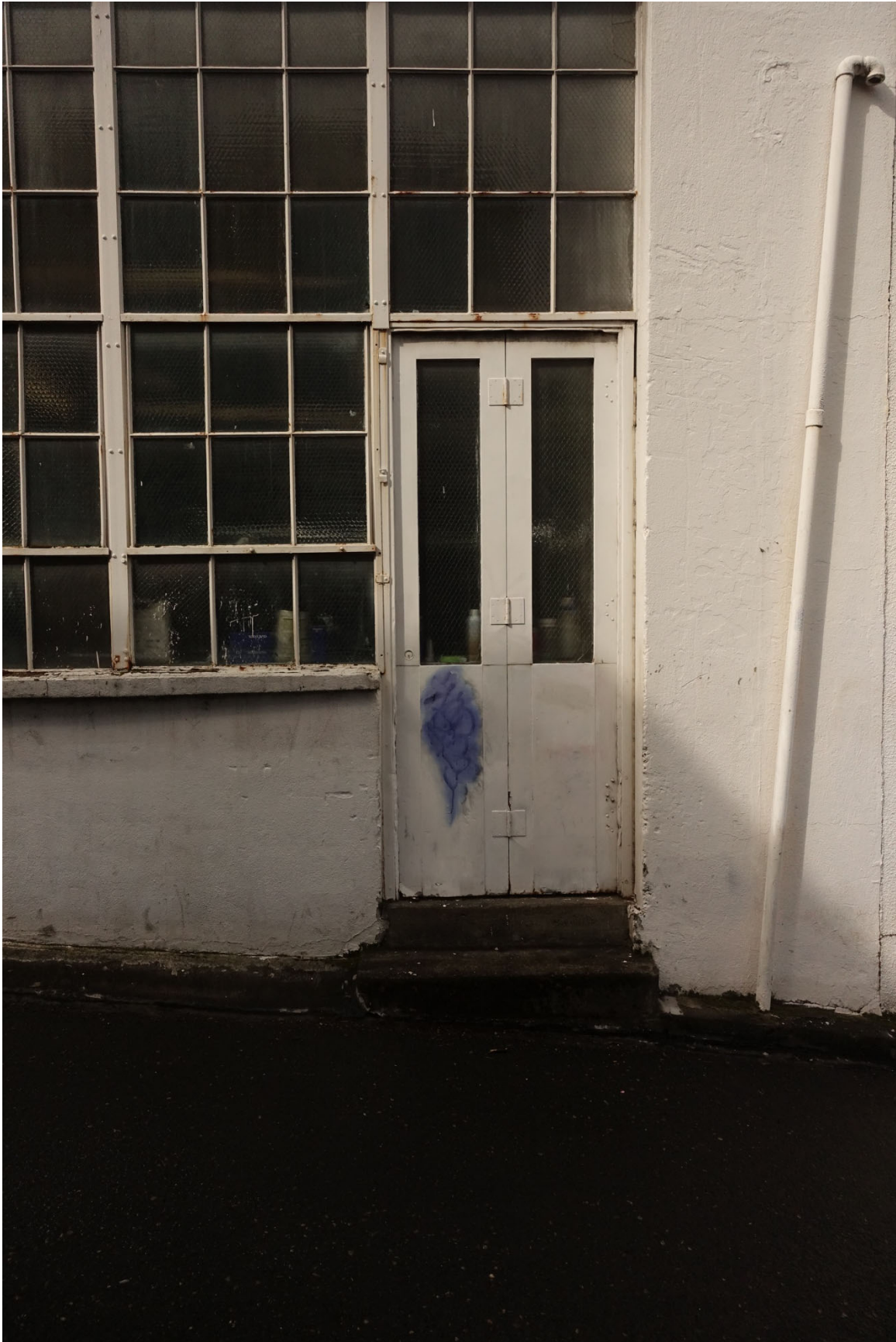
Photograph 12 of 12: OR_Multnomah_CoveyMotorCarCompany_0012 Detail of riveted metal window mullions, awning window opening, patterned glass windowpanes, and accordion door.
